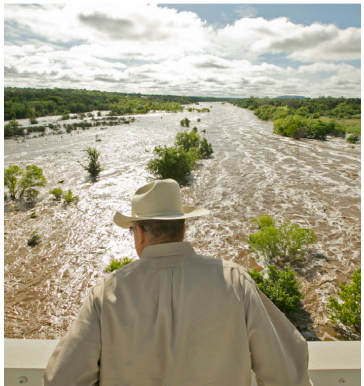
▲ Top: Flooding in Los Fresnos. Bottom: Flooding on Llano River.
