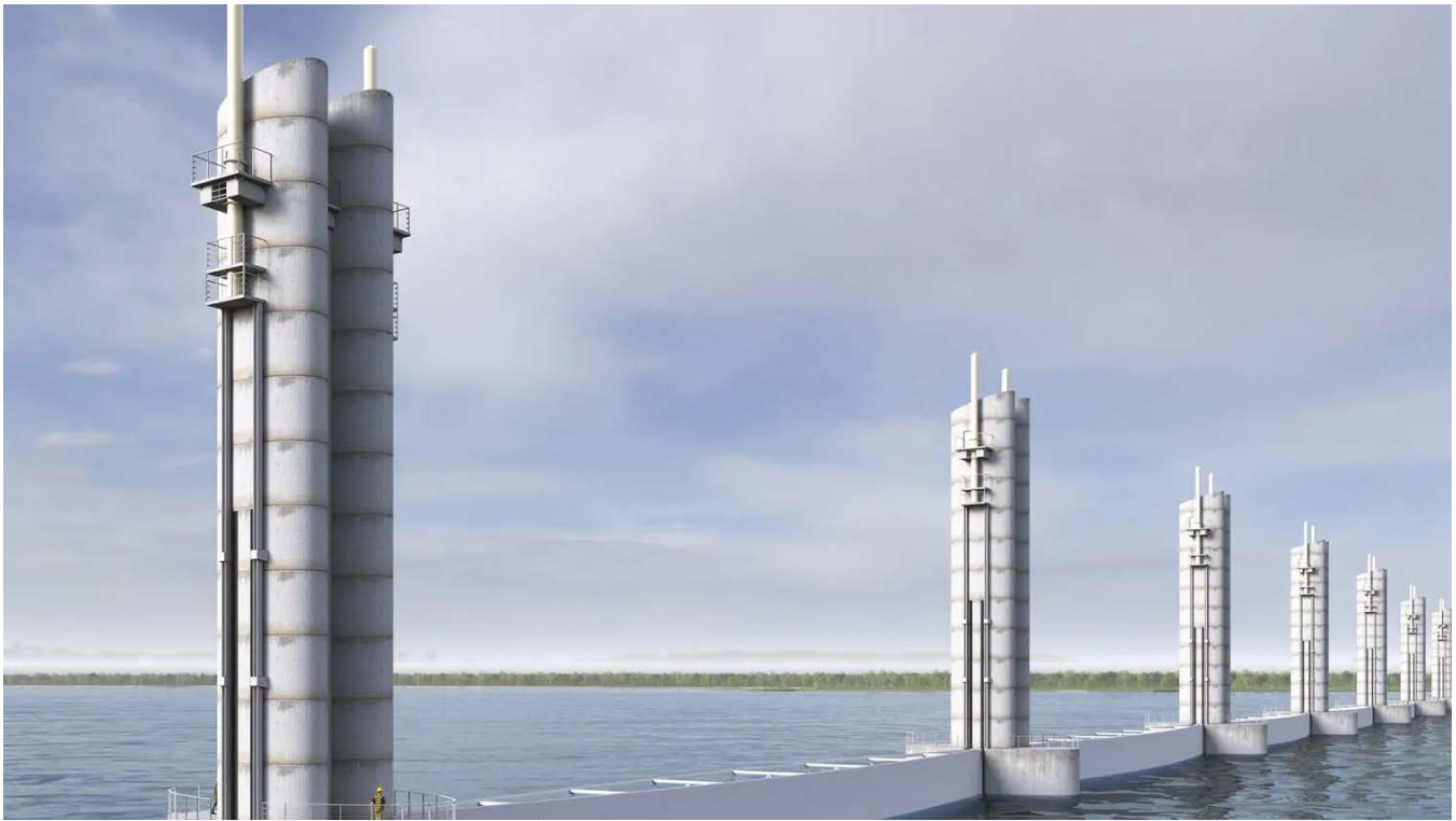
Illustration of vertical lift gates proposed in the Coastal Texas Study (US Army Corps of Engineers)
