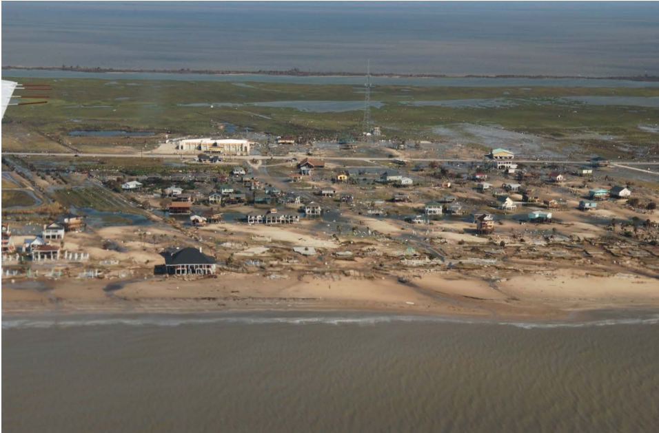
Damage caused by Hurricane Ike in 2008 (United States Geological Survey / Karen L.M Morgan)
